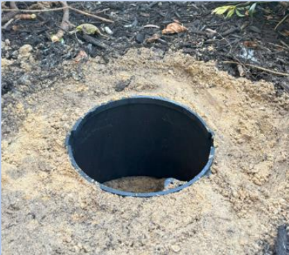
Pack dirt around UP1001
